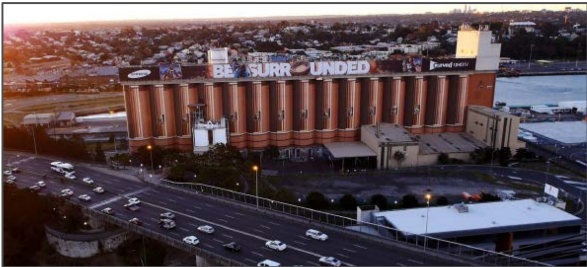
Figure 2 | Southern elevation of silos with existing signage (Source: Applicant)
