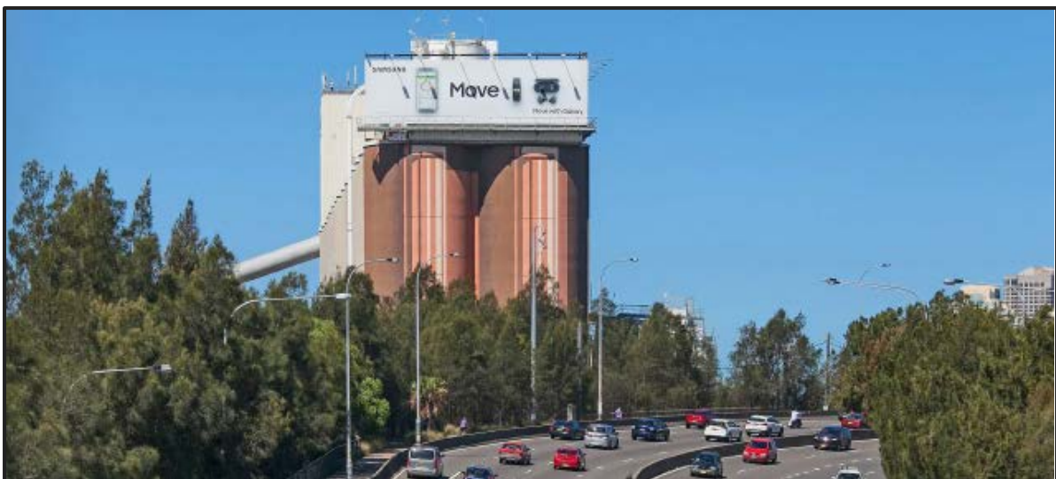
Figure 3 | Western elevation of silos with existing signage (Source: Applicant)
